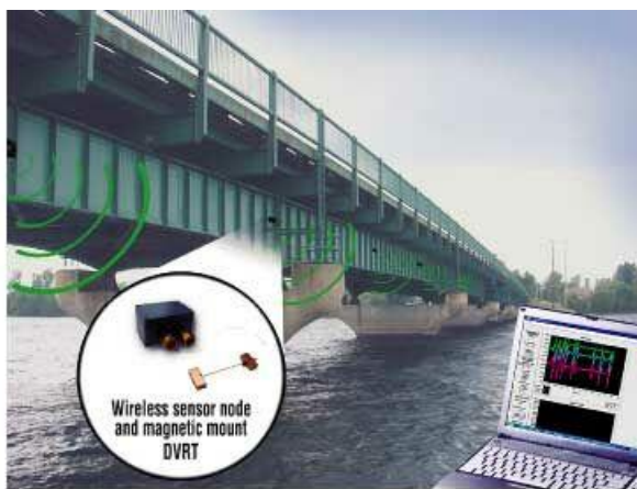
3. Wireless sensors are used to measure long-term stress and strain in civil engineering structures like buildings and bridges. (Courtesy: Microstrain Inc.)
